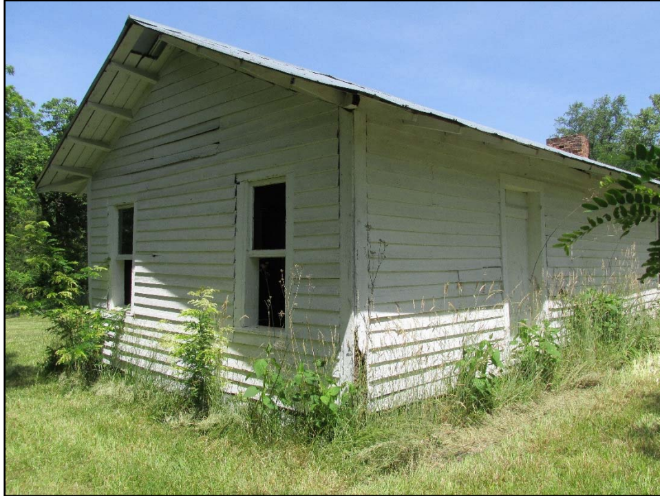
Figure 11. South and east elevations, original batten door.
