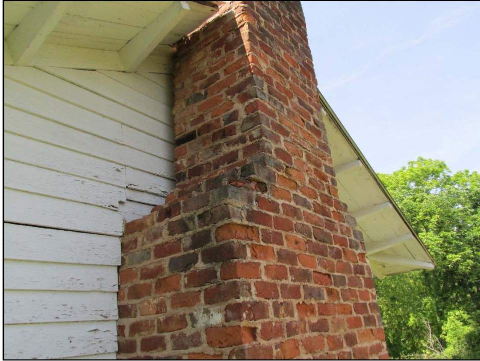
Figure 6. Brick chimney on exterior of north elevation; also tapered rafter tails.
