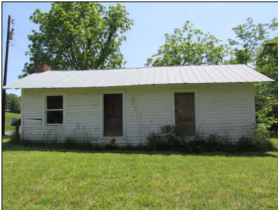
Figure 10. West elevation of Reeves Kitchen and Dining Room, replacement doors.
