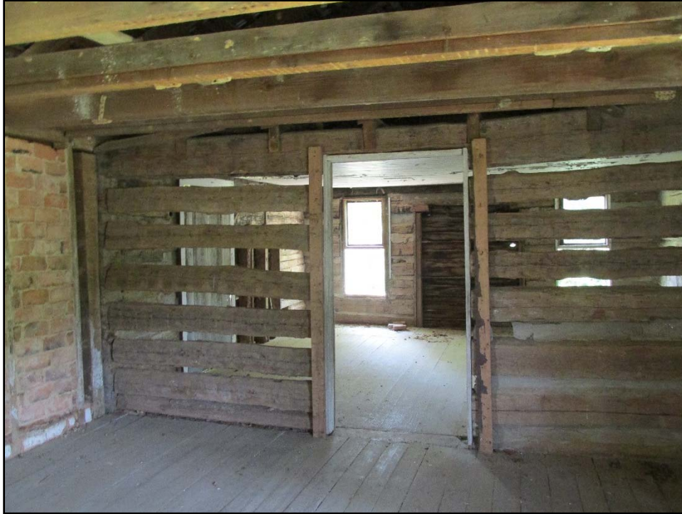
Figure 8. Reeves Kitchen and Dining Room, from frame addition toward original log single pen, with former chimney location visible on far wall.
