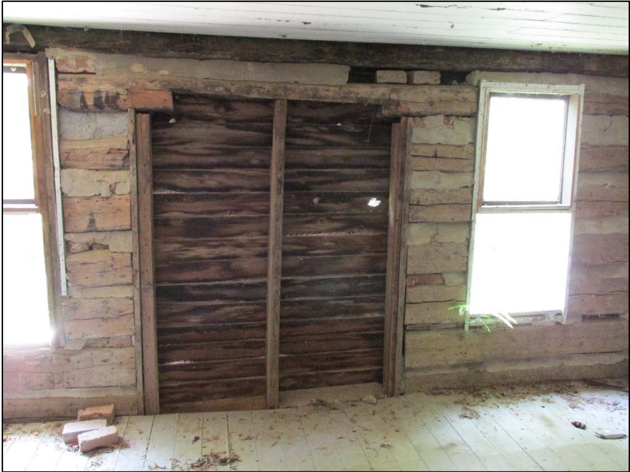
Figure 14. Interior of original room: wall construction and former chimney location.
