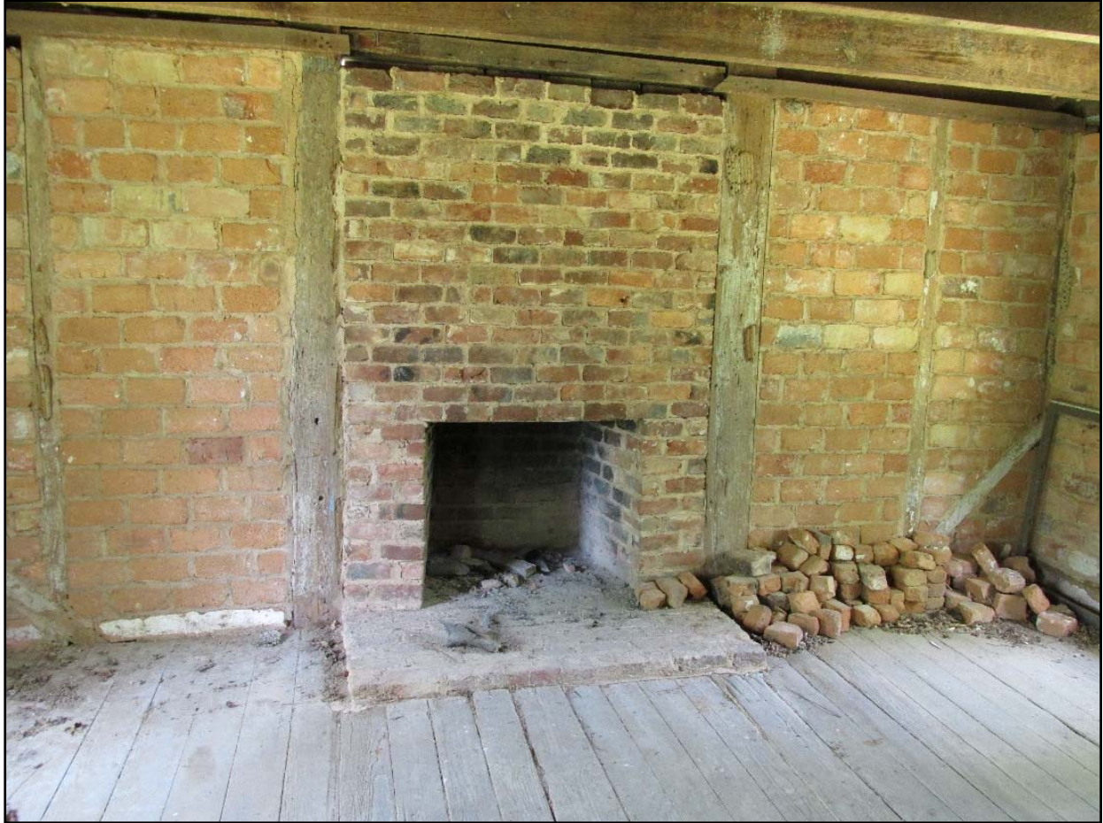
Figure 13. Interior of timber frame addition: fireplace and brick nogging.
