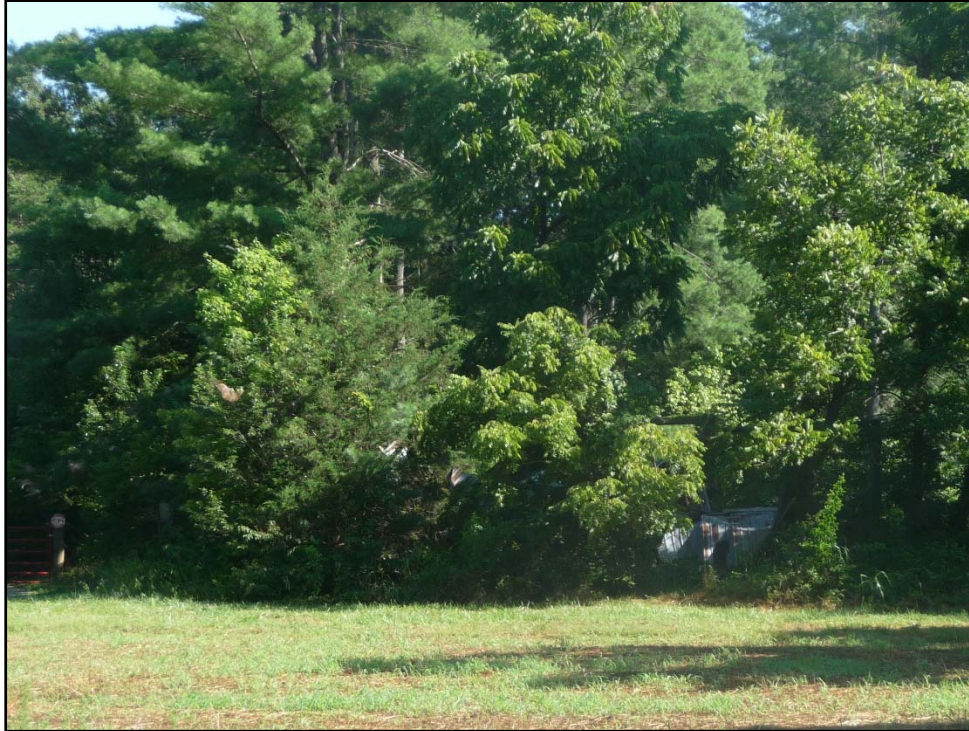
Figure 25. Current condition of Holder-Shore House.
