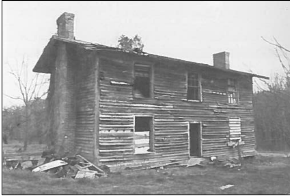
Figure 27. Former appearance of Smith House (Phillips 1987:260).
